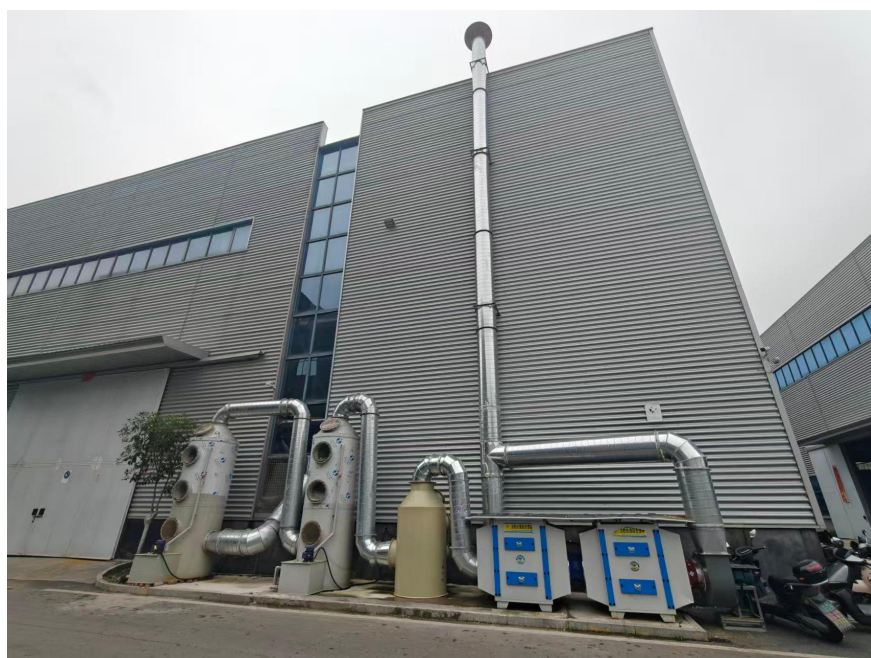
“喷淋净化塔+干式过滤+二级活性炭吸附”+DA002 排气筒
